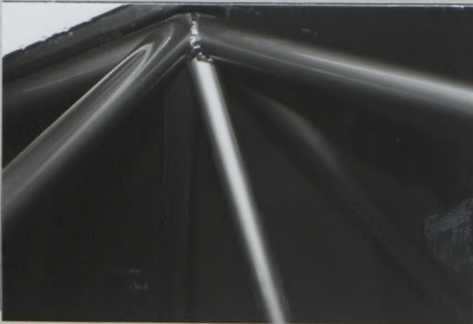
PHOTO No. 9 (REAR SUPPORT BARS TO STRUT TOWER)
