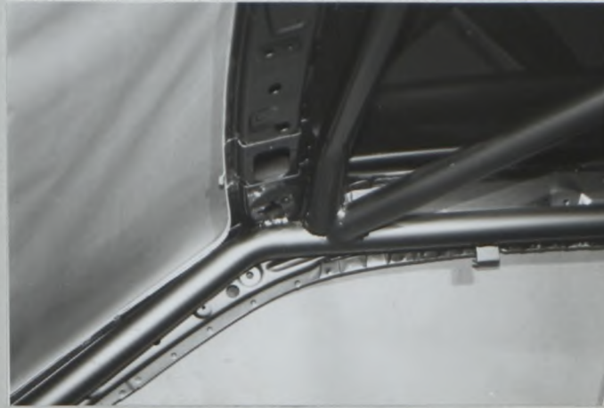
PHOTO No. 4 (FRONT ROLL BARS TO A-PILLAR AND ROOF)
